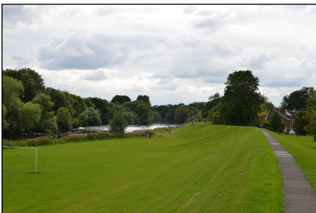
Flood defences at Neasham
